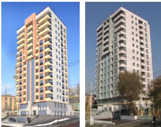
Fig. 2. Design view of the 17-story base isolated apartment building “Sevak” constructed in Yerevan and its current view
