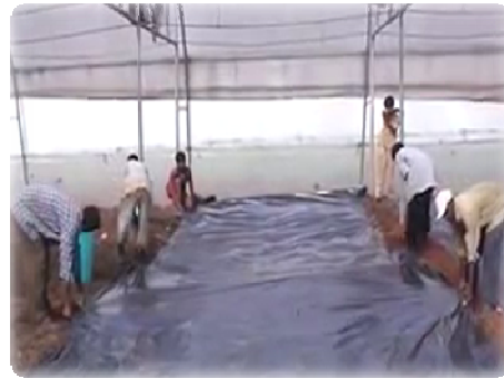
Fig: 2b. Polyethylene Sheet Covering
