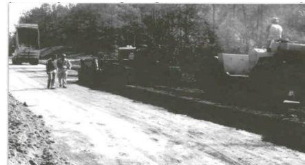
Figure: Cement treated fly ash base course
