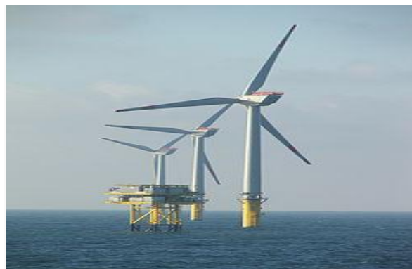
Fig.4.1 Wind turbines and electrical substation of Alpha Ventus in the North Sea
