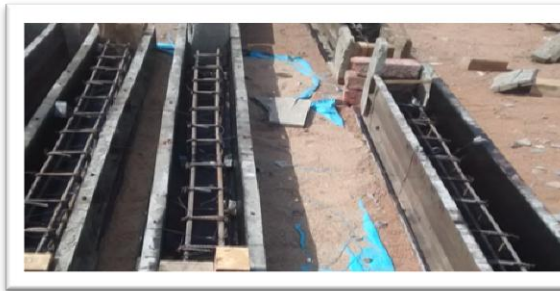
Casting of test beams:
