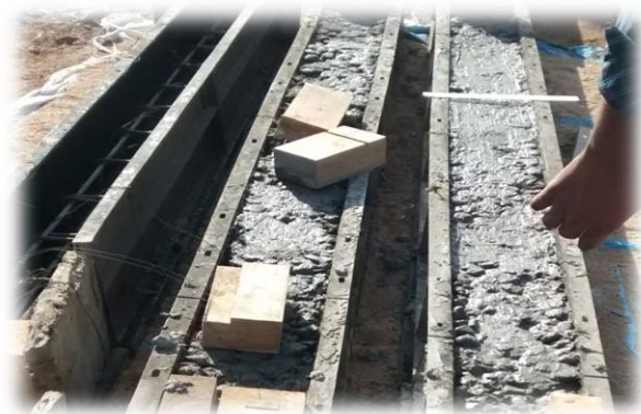
Compaction and casting
