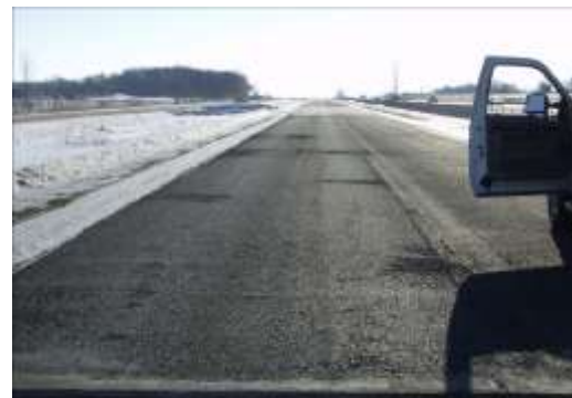
Final Porous Pavement
