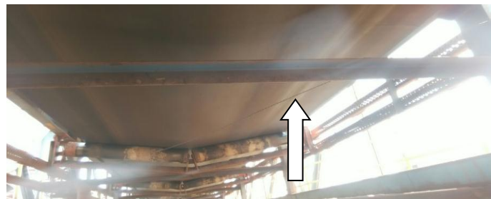
Fig.7 After laying LHS Cable
