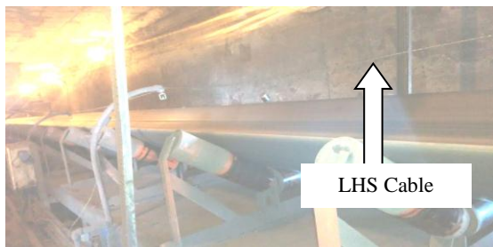
Fig.6 After laying LHS Cable
