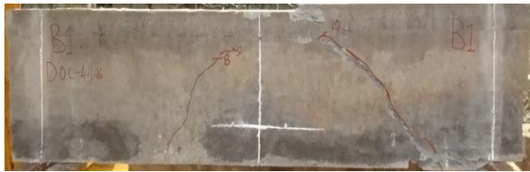
Fig. 5.4 Modes of cracks for B1 at failure
