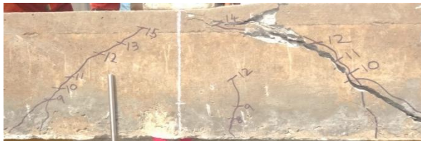
Fig. 5.6 Modes of cracks for B3 at failure
