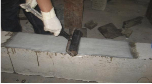
Figure 3.4 Application of epoxy and hardener on the beam
