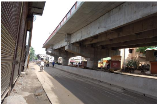
(Fig 2). Existing Site Bridge Remaining from Railway Crossing
