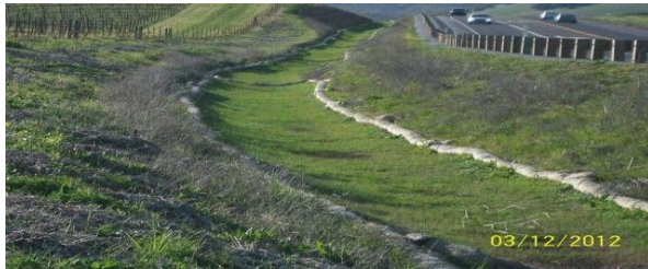
Figure 7 Steep-Sloped Channel with Composite Vegetative Lining
