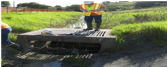
Figure.2 Roadside Channel Outlet to Storm Drain at Drop Inlet
