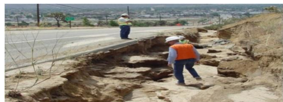
Figure.3 Damaged Channel
