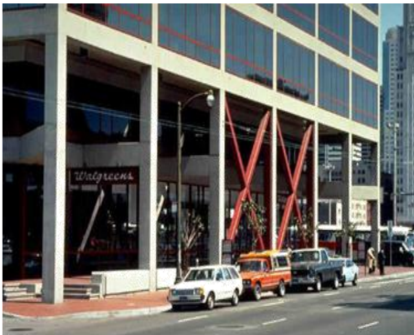
Steel bracing in RC frame
